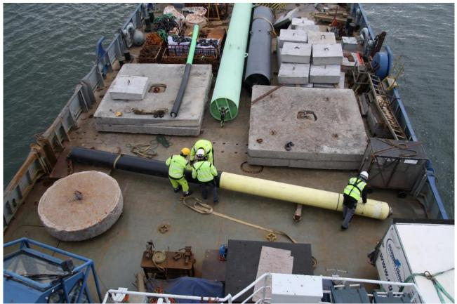
Figure 5. Preparation of moorings on board the buoy tender vessel "Seili". Picture Seppo Virtanen / SeaHow
